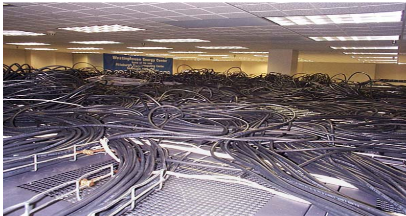
Figure 2. Centralized federated switch cabling for 750 node cluster
