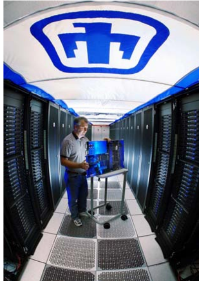
4500 servers, Mellanox InfiniBand interconnect 53TFlops, 84.66% Linpack efficiency
